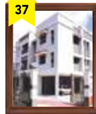
BLOSSOM APARTMENTS Sakthan Thampuran Nagar, Trichur
